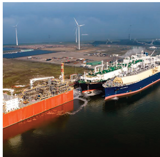
The Eemshaven LNG receiving terminal is being expanded
