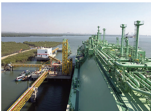
Pakistan's LNG import terminal at Port Qasim, Karachi
