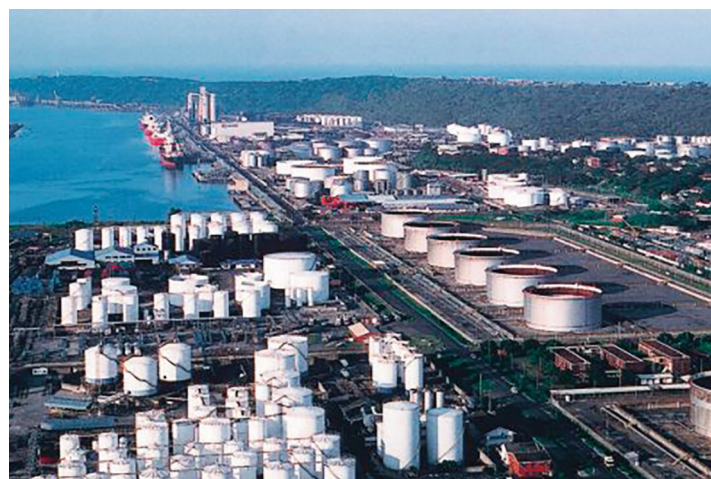
Vopak's Zululand Energy Terminal at Richards Bay
