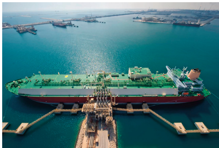
LNG carrier docked at a loading terminal at Ras Laffan
