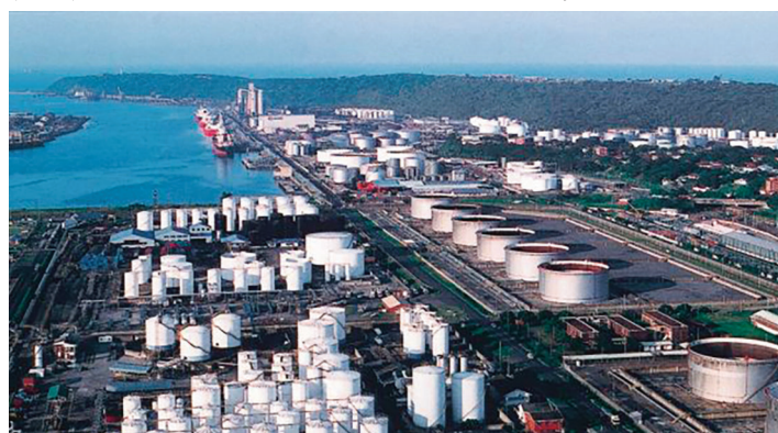
Vopak-led Zululand Energy Terminal
