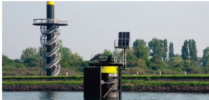
Paal 83, mooring post installation
