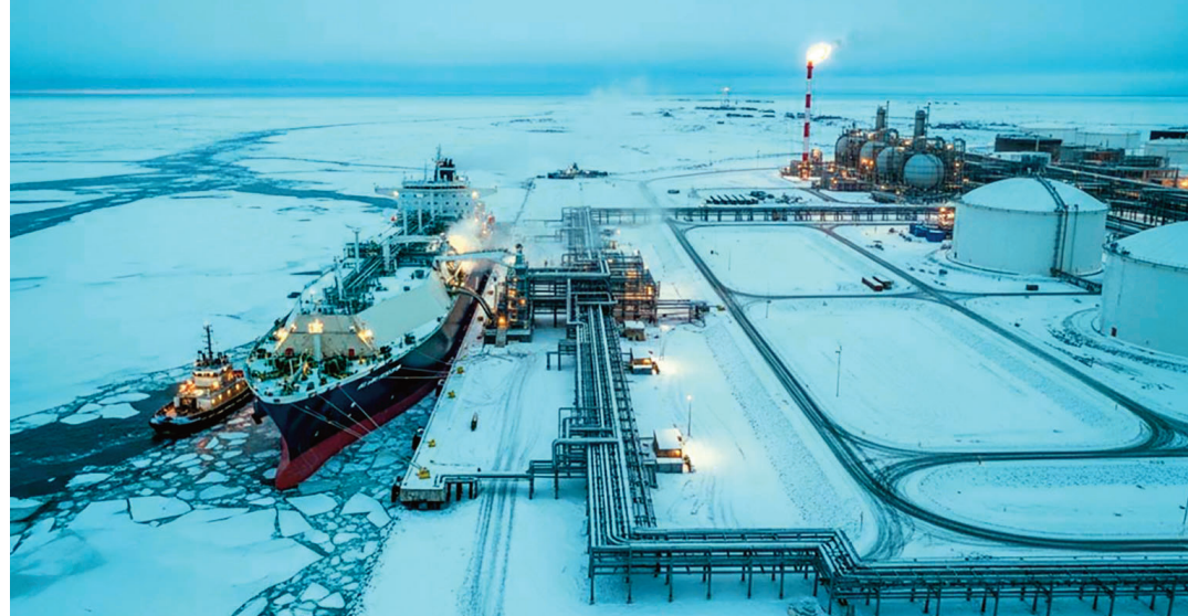
Ice-class tanker berths at Novatek’s Arctic LNG 2 terminal
