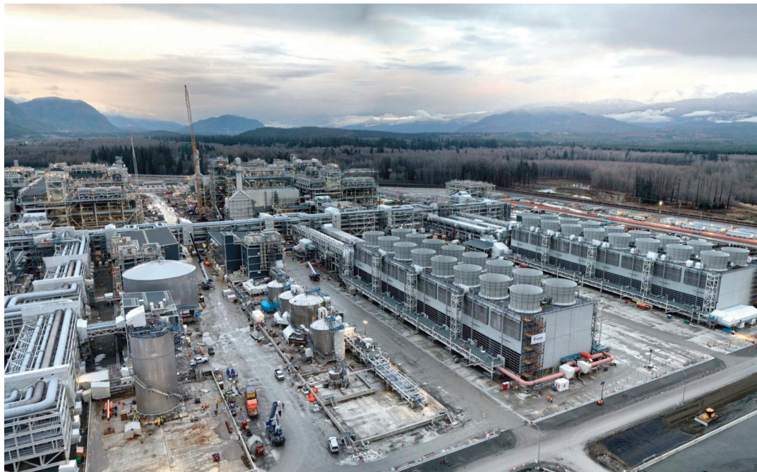
Construction is progressing at LNG Canada terminal, Kitimat
