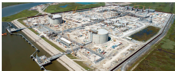
Calcasieu Pass LNG terminal will start operations in under 68 months from taking FID
