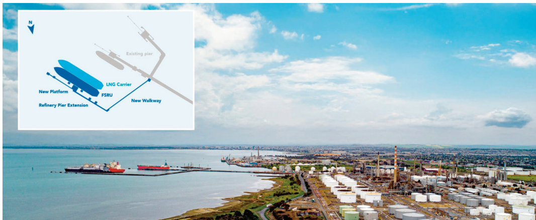
Geelong's energy hub
