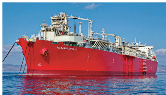
The Alexandroupolis FSRU terminal
