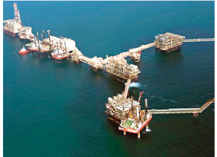
ADNOC Gas' Das Island facility
