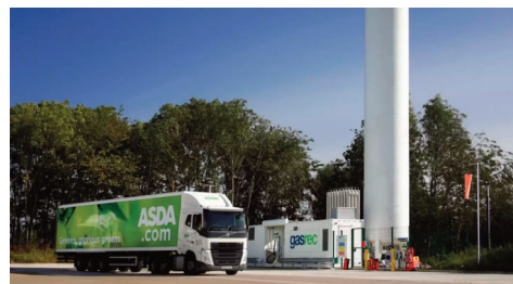
ASDA bioLNG refuelling facility
