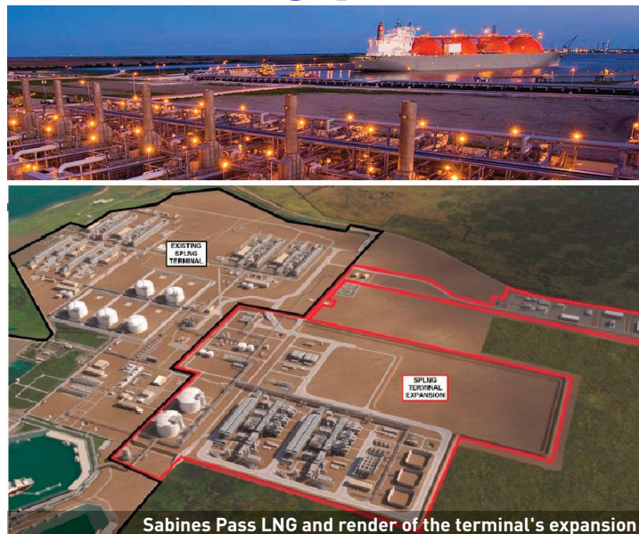
Sabine Pass LNG and render of the terminal's expansion
