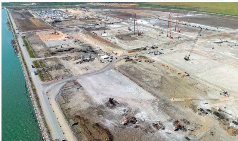
Construction-progresses on Sempra's Port Arthur LNG terminal
