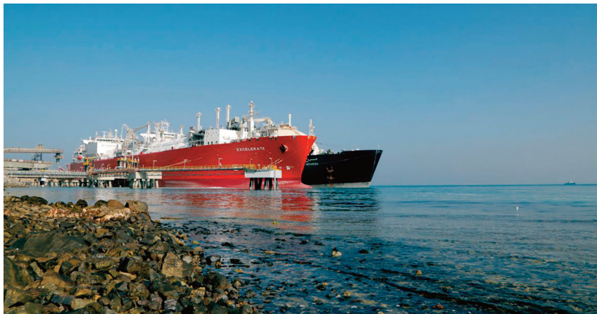
The original Ruwais FSRU terminal
