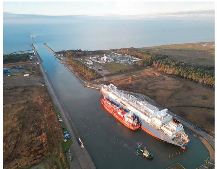
RWE's Mukran LNG terminal has received another two permits
