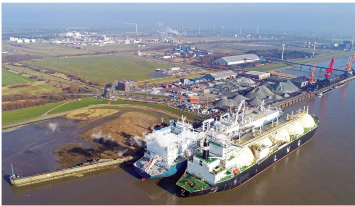
DET has taken control of the Brunsbüttel LNG receiving terminal
