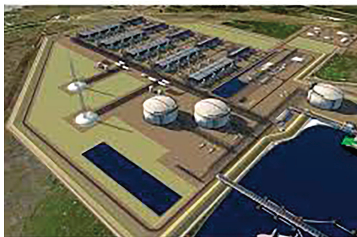
Bechtel has been re-assigned the EPC contract for Louisiana LNG, formerly Driftwood.
