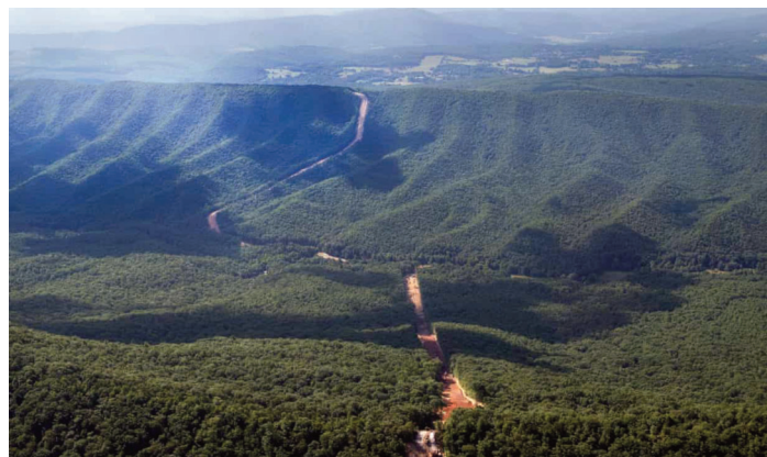
The Mountain Valley pipeline at Brush Mountain in Virginia
