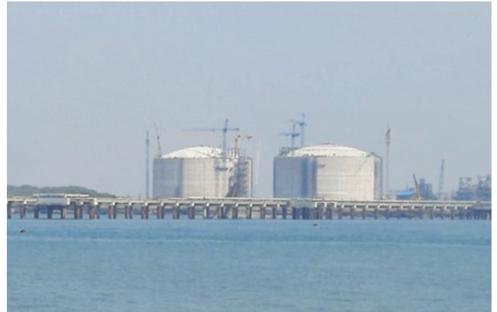
Hindustan Petroleum's new LNG facility Gujarat state
