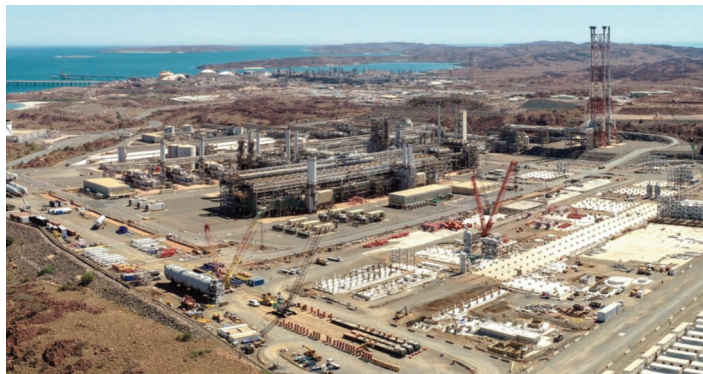
The Pluto LNG plant is having a second train constructed
