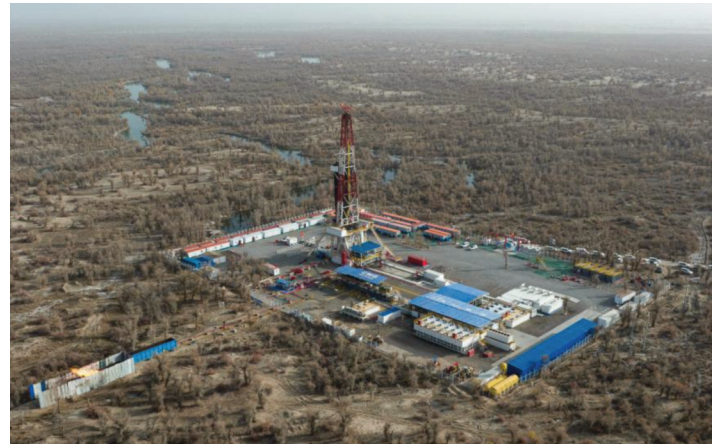
Sinopec has been increasing exploration and production
