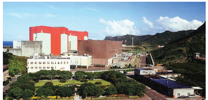
Guosheng nuclear power plant on the coast in northern New Taipei
