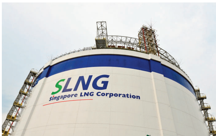
SLNG storage tank
