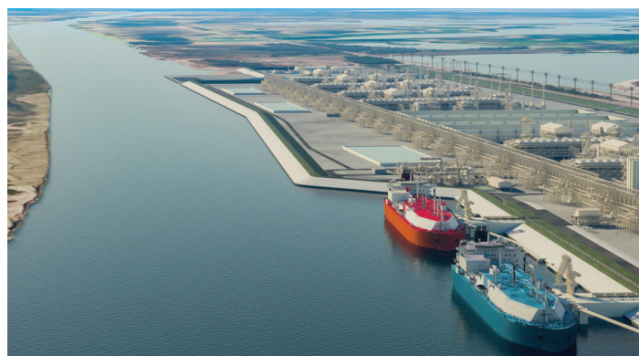
Render of Rio Grande LNG at the Brownville Ship Channel
