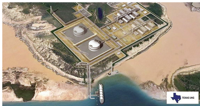
Render of Texas LNG on the Port of Brownsville
