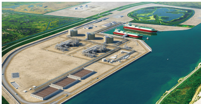
Port Arthur LNG is one of three projects to take FID so far this year
