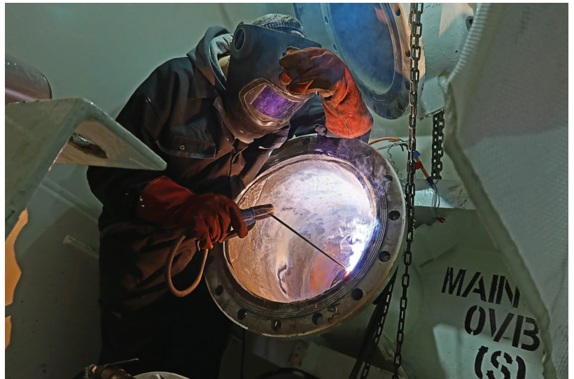
Hydrex has completed scrubber pipe repairs on two LNGCs
