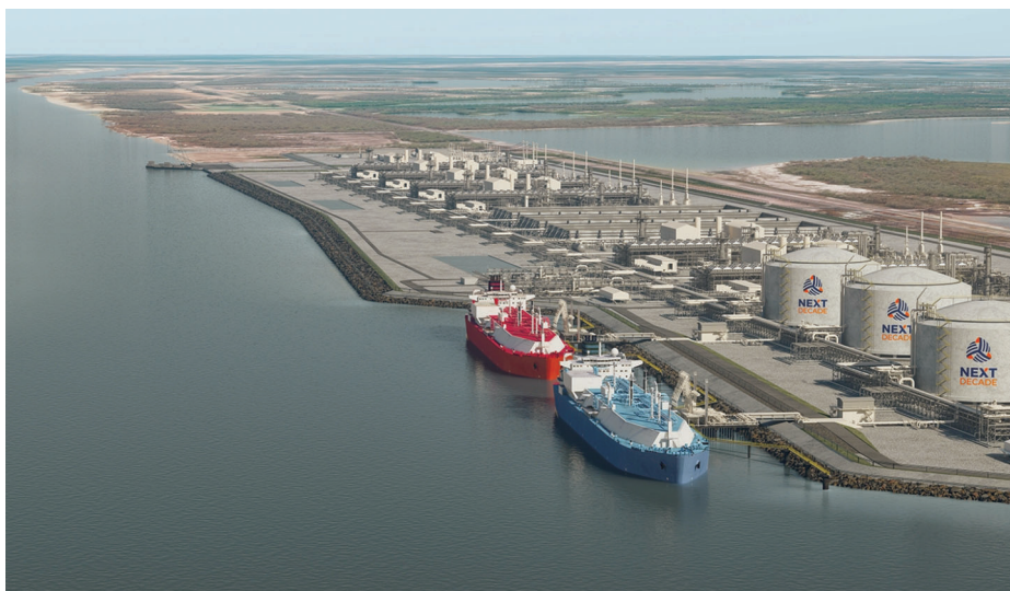
NextDecade's proposed Rio Grande LNG terminal
