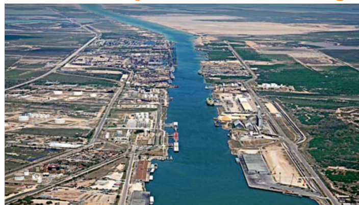
The Rio Grande LNG export project site on ship channel
