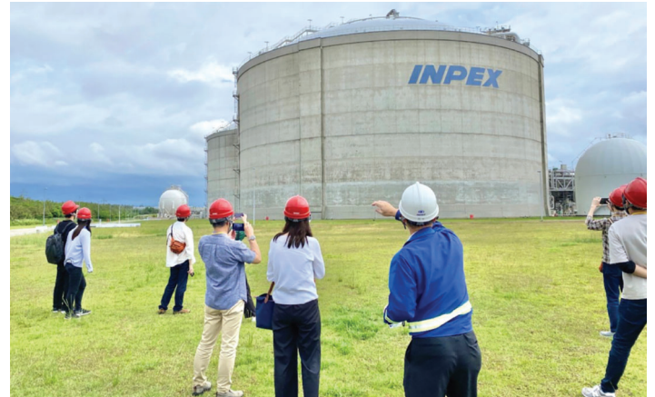
LNG tanks were popular with visitors for photographs
