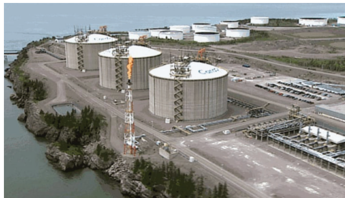
St John LNG terminal with storage capacity of 480,000 cubic metres in three tanks started up in 2009
