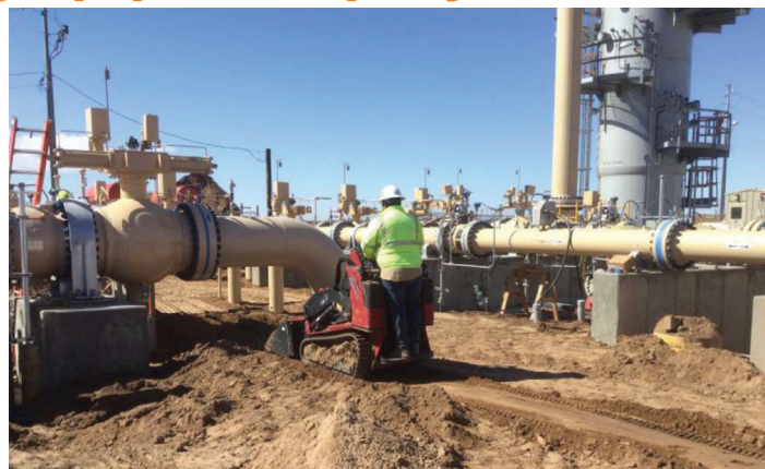
View of El Paso Meter Station as crew backfill newly installed pipe for US project pointing to Mexico
