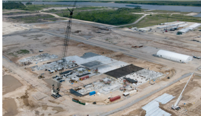
Driftwood LNG construction underway managed by Bechtel
