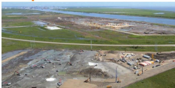
Civil construction has started at the Port Arthur LNG site
