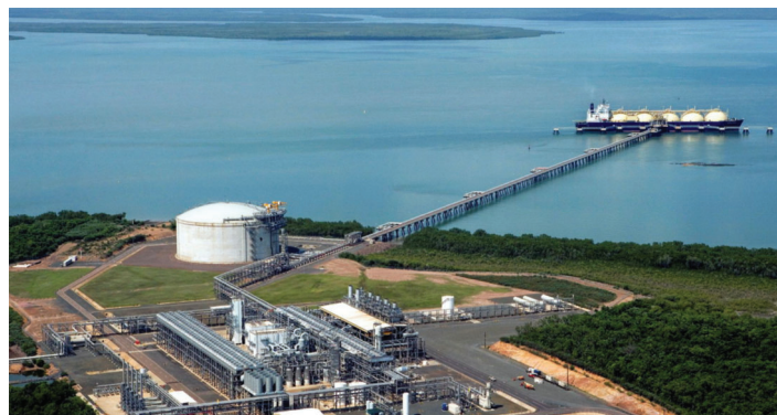
Darwin LNG plant now awaits start-up of Barossa gas field
