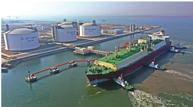
Sinopec unloads a Q-Max LNG tanker at its Tianjin regas terminal
