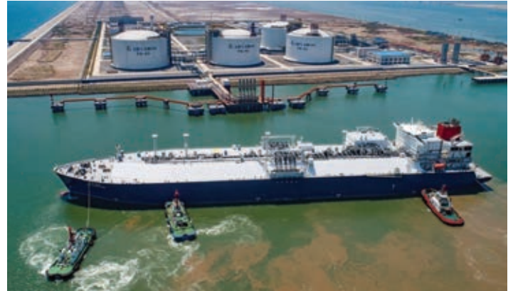
LNG tanker arriving at Tianjin regas terminal, operated by Sinopec.
